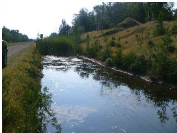
South Railway Ditch
